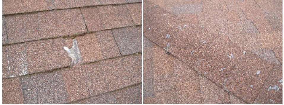
Damaged shingle and popped nails
